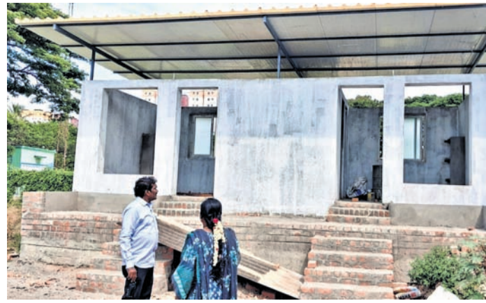
Lounge room work for conservancy workers under way in Manali | EXPRESS
