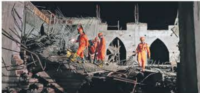
The church was under construction for past eight months | SOINESH
